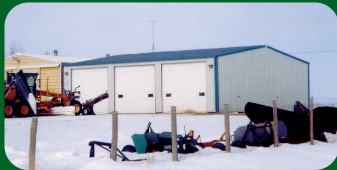
■ R.M. maintenance shop
