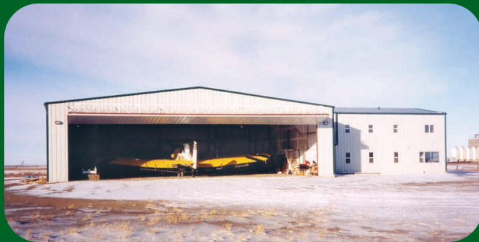
■ airplane hangar / office
