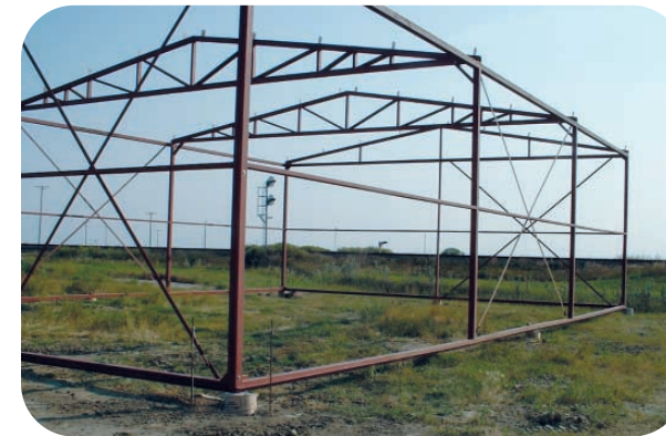
■ base tube on concrete pilings
